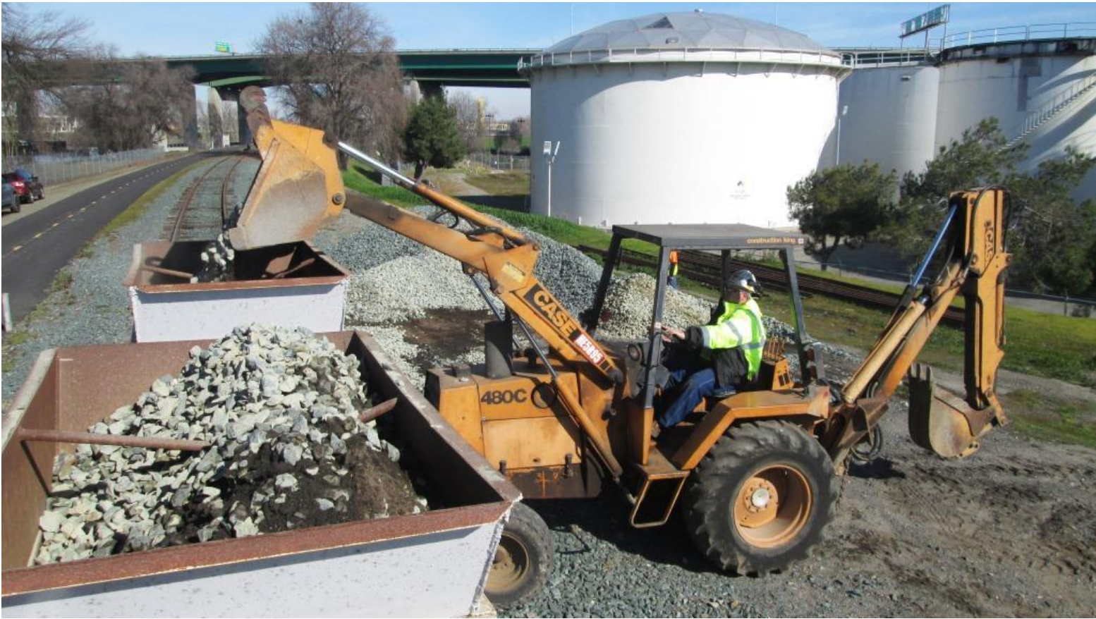
A more dramatic view of Mike F. loading rock into the hopper-cars
