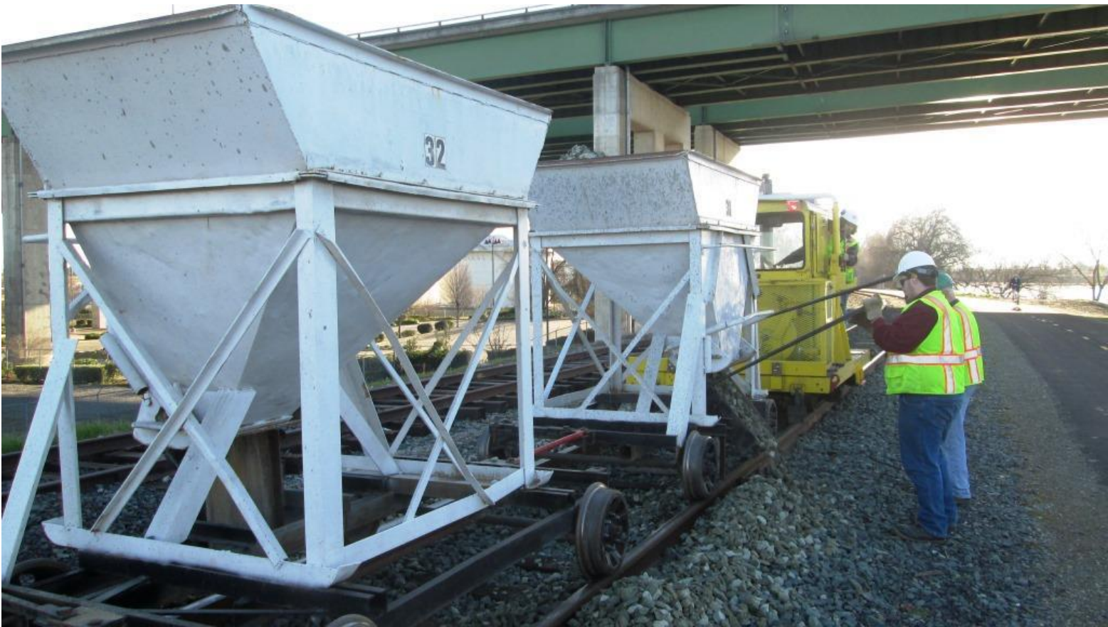
Josh and Tom continue with the ballasting of the track in the afternoon
