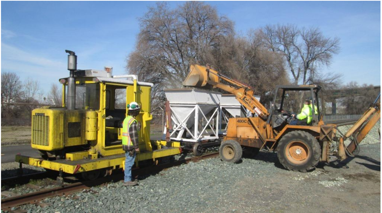
With the presentation done, Mike F. on the back-hoe loads the side-dump hoppers
