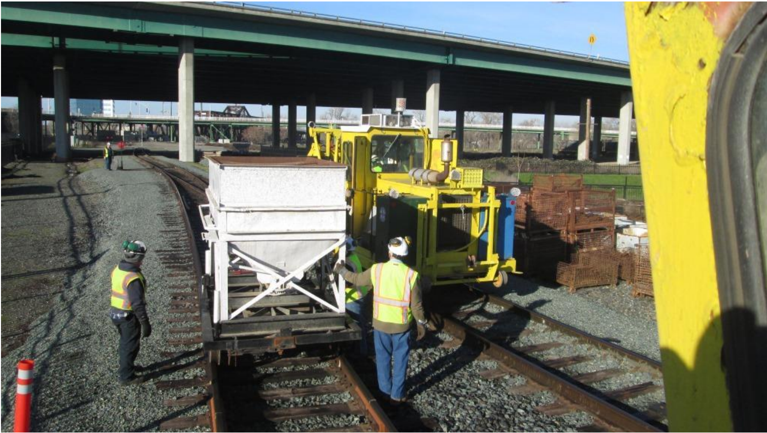
Heather brings forward the tamper which has now been designated to pull the hopper-cars
