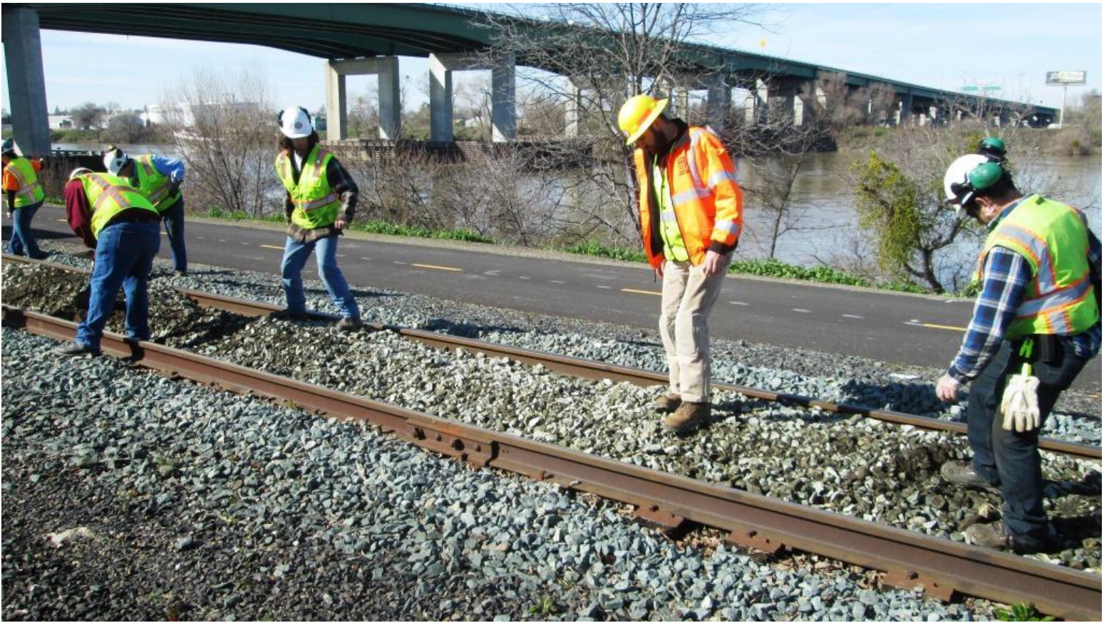
Matt, Chris M., and Joe knock-down high-spots and spread the rock by stomping on it
