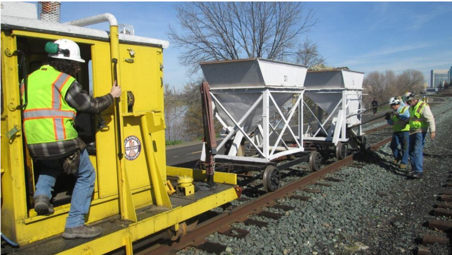
With Matt at the controls of the Kalamazoo creeping south, Alan and Clem disgorge rock along the line
