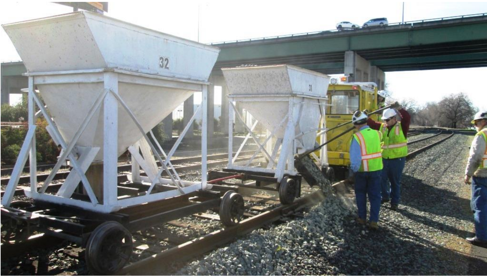
Clem and Josh pour ballast-rock onto the opposite side of the track
